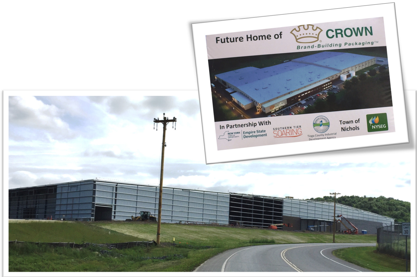
Crown, Cork & Seal aluminum beverage can manufacturing facility in Nichols
