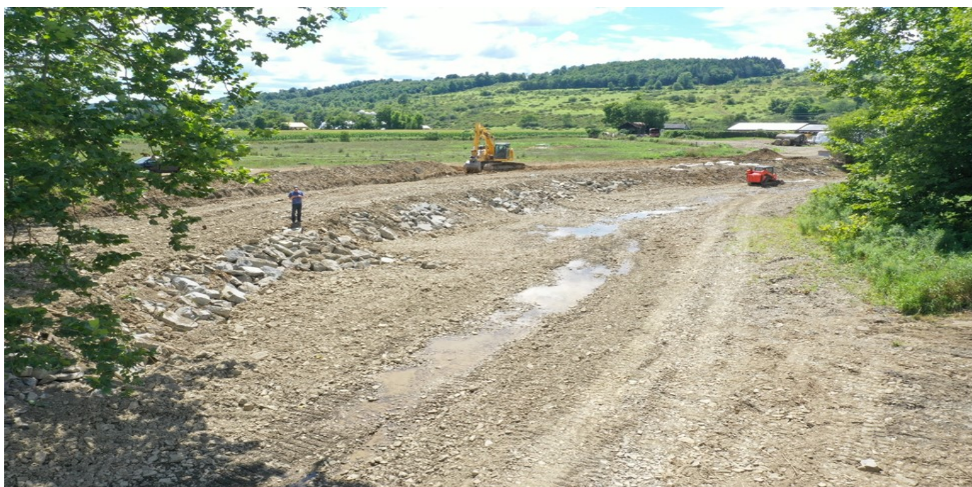
Above: USC Wetland Team working on streambank stabilization
