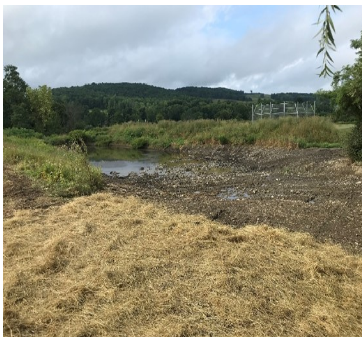
Above: After sediment was removed at SVE basin
