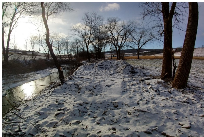
Above: Removal of berm along Little Nanticoke Creek
