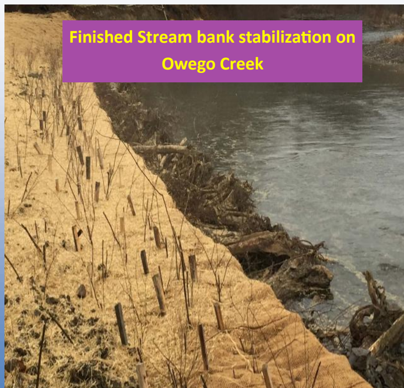
Live Willow Stake bank installation on Susquehanna River
