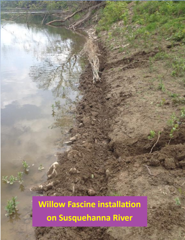
Live Willow Stake bank installation on Susquehanna River
